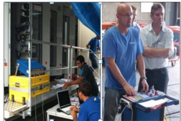
Figure 8: CMC test on site (left). Primary test with CPC (right)
