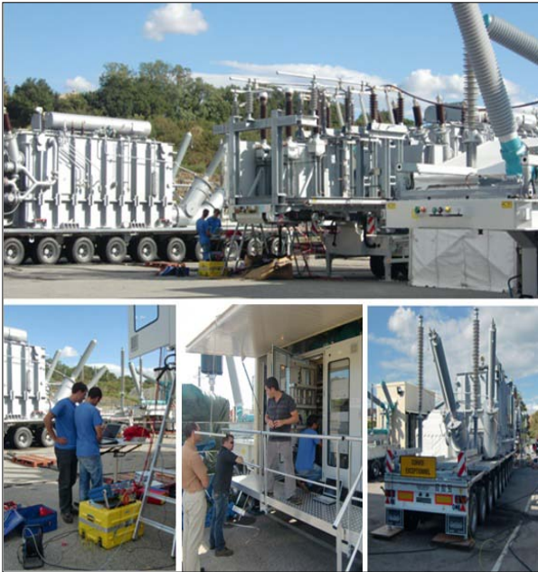
Figure 11: Commissioning of 220 kV GIS mobile substation
