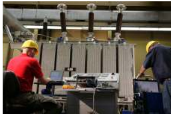
Fig. 13. PD test on transformer, 30 MVA 115 kV
